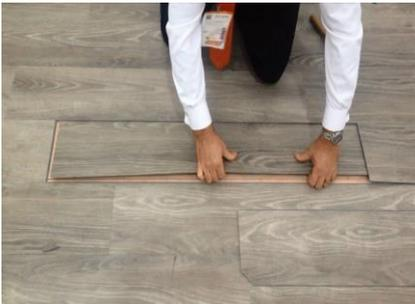
5. Slide the replacement plank under the male side end of the adjacent boards and lower the plank (male side end) into the female groove of adjacent planks ready for installation.
