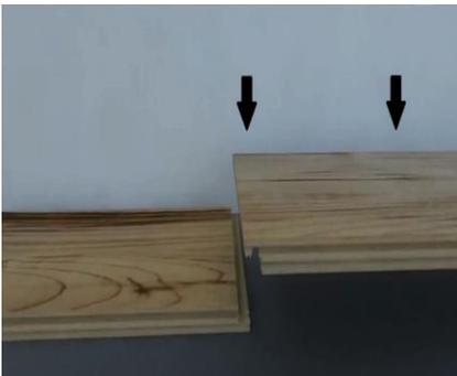
3. Lay the male side of the adjacent plank into the end of the female track. When lowering the tile into place the product will self-align into the track. Once placed, simply use a swinging motion with your foot slightly across the planks to install. A rubber mallet may be used with a similar motion to assist with any stubborn or high areas.
