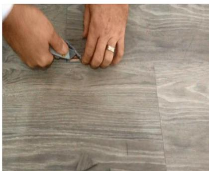
2. Use a small flat head screwdriver and tap out cut corner piece, which has been cut.
