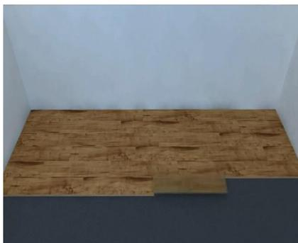
8. To fit the last row, start by using the offcut piece from the previous row. Lay the plank on top of the previous row. With the male joint to the wall, use a ruler to draw a cutline. Don't forget to allow room for spacers. Cut the plank and attach into position.
