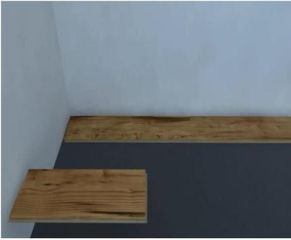
5. Begin the second row with the offcut piece from the first row to stagger the pattern. Pieces should be a minimum of 150 mm (6") long. Remember to use spacers along each wall to maintain an expansion space of 8 - 12 mm (3/8" - 1/2") between the wall and the flooring.
