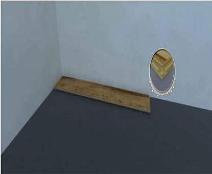
2. Start in a corner by placing the first plank with the male side facing the wall. Use spacers along each wall to maintain an expansion space of 8 - 12 mm (3/8" - 1/2") between the wall and the flooring.
