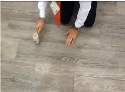
6. Use a mallet to re-engage all edges until new plank is installed and flush.
