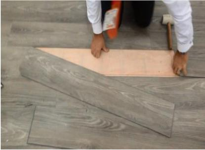
4. Use your finger to simply run along the partly disengaged plank, inverting both edges as to not damage the adjacent planks. Remove damaged plank, clean subfloor free of all debris.
