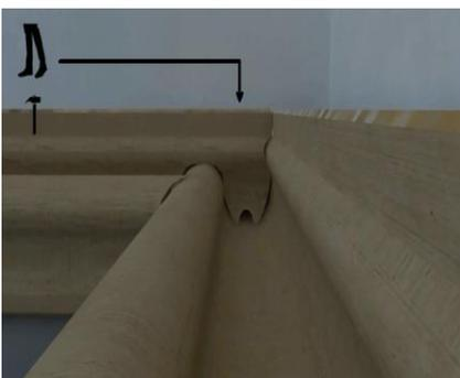
To attach the second row to the first row, kick the male side into the female side of the first row vertically. Continue laying remaining rows in this manner.
