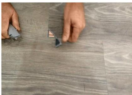
1. Carefully cut a corner of the damaged LVT plank. Diagonal (as shown in the picture) with a utility knife (cut five times or more until the plank is penetrated to the subsurface).
