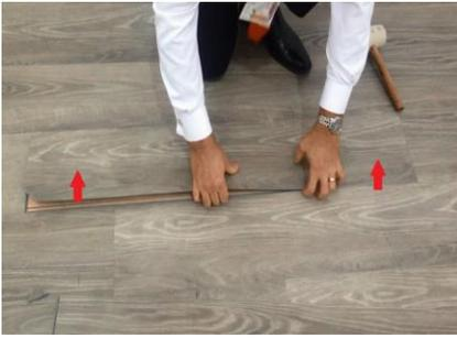
3. Use the screw driver to simply pry the edge of the cut corner out.
