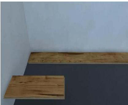
6. To start your second row, lay your first plank on the subfloor. Take your second tile, engage and lock into the end female of the first tile vertically. When knocked by a rubber mallet or stepped on, the tile will engage and lock into place with light pressure or kicking. The planks should be flat to the floor. Make sure planks are fully engaged with no gaps between planks on sides or ends. Continue assembling the planks this way until you have your second row complete.
